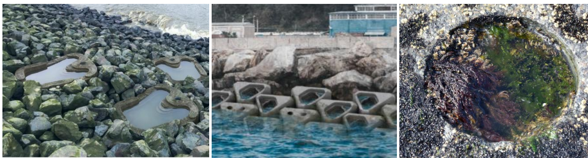
Figure 4.5: Photo of ECONcrete tide pools (left), artist impression of ECONcrete Coastalock (middle) and photo of drilled rock pool (right) (source: EOS Ecology)
